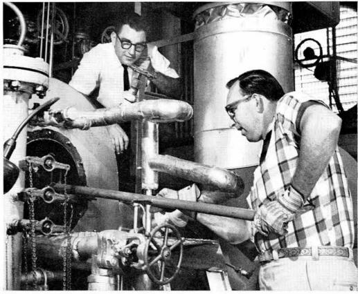
OPERATION OF NEW TOOL for removing steam boiler manhole covers is checked by designer N. N. (Norm) Sirnic (8254) while J. R. (Rudy) Grund (8222-1) removes a boiler cover located two feet inside the circular opening shown. Tool eliminates the need for struggling with a 68-pound cover in cramped quarters during boiler inspections.
